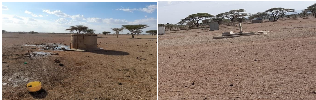
Plate: 1 Community water point and manual water pump
